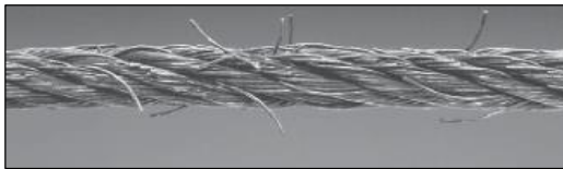
Cable with Corrosion
